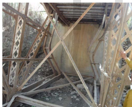
End members before Retrofitting
