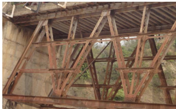
Figure 2: Side View of 40 m steel truss bridge
