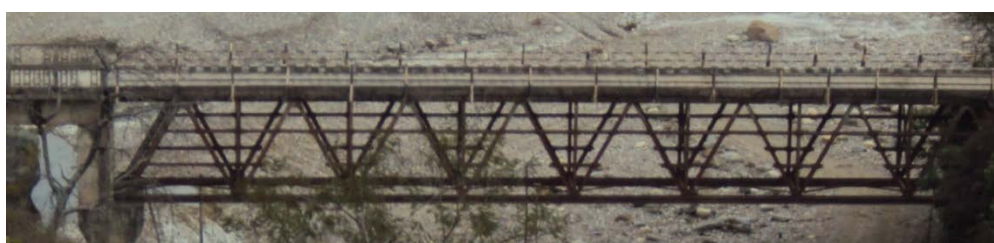
Figure 1: 40m span Steel truss bridge in HP India
