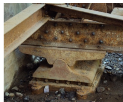
Bearings after retrofitting
