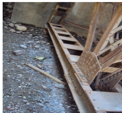
Bottom members after retrofitting
