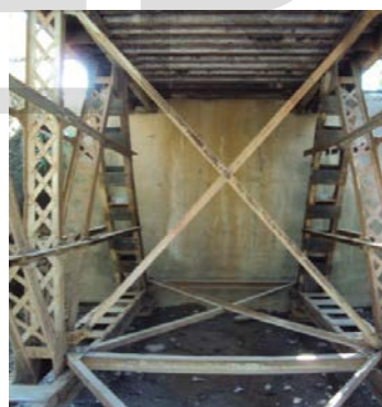
End members after retrofitting
